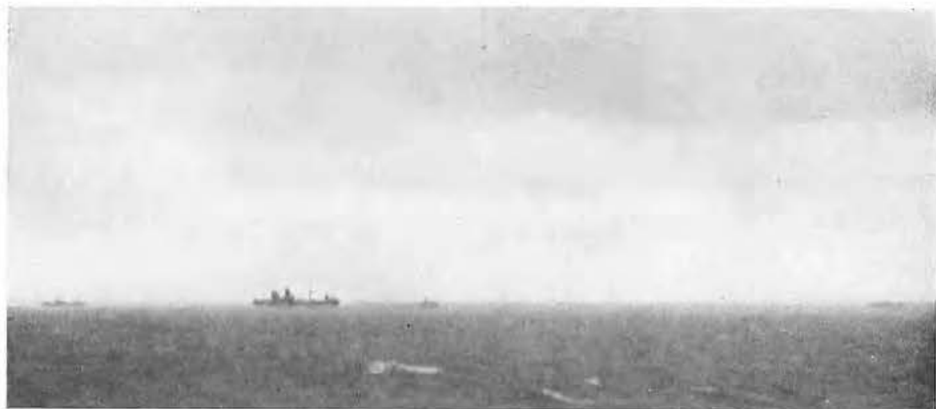
FIG. 29.—Our latest mines cannot be disposed of with safety even by the sperrbrecher . This photograph, taken off Terschelling by a Beaufighter of Coastal Command, shows one of the most notorious sperrbrecher , "A.E." (5,000 tons), being towed stern first, the whole forepart of the vessel having been blown off by a mine. (Compare the silhouette.) This ship used to escort merchant convoys on the Cuxhaven-Rotterdam route, and such serious damage to these anti-mine ships directly benefits our minelaying campaign. (See page 13.)
