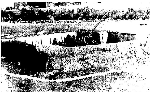
Dummy A.A. Post. Constructed by means of sandbags (empty). Dummy tracks and spoil can be seen in the photograph.
