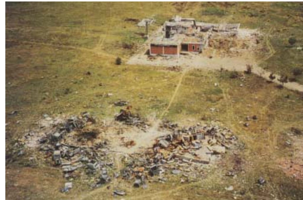
A radio relay station destroyed by Nato air strikes.
