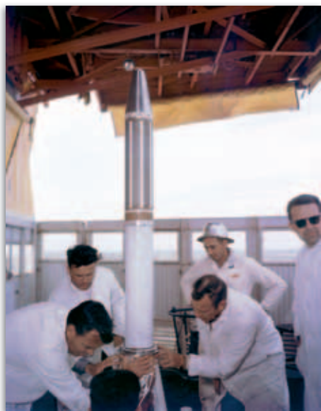
Installation of Explorer 1, the first United States' satellite, to its launch vehicle, Jupiter-C, January 1958.
