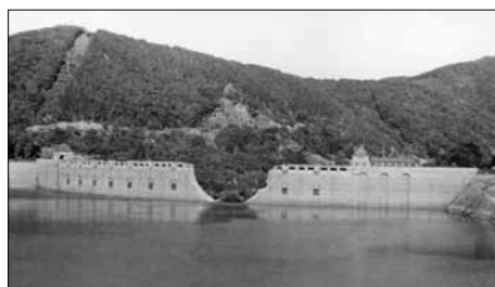
German photograph of the breach wall of the Eder dam
